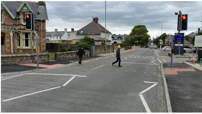
Pedestrians using the operational controlled crossing over the A82 at Smith Avenue
