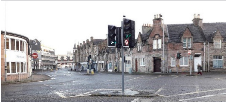
Kenneth Street Tomnahurich Street Junction: Image showing the central island which is planned to be removed.
